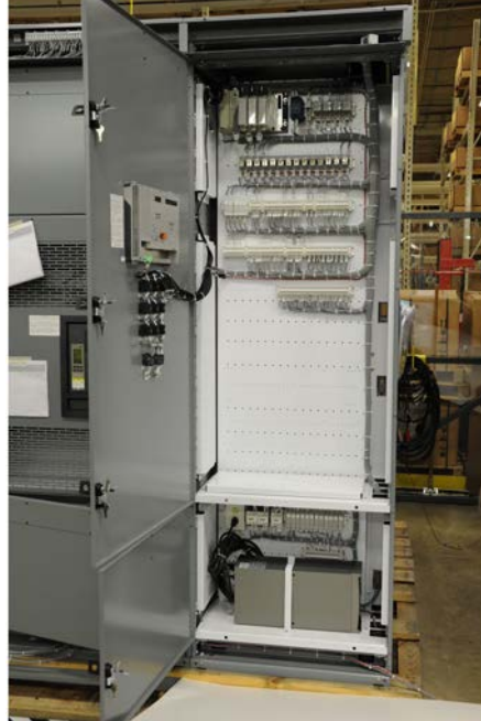
Figure 15 - Auxiliary Section
