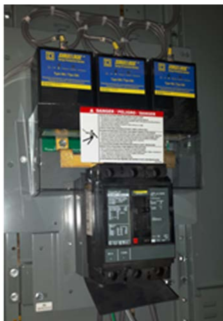
Figure 66 - Surge Protection Device (SPD) in rear cable compartment sidewall of Rear Accessible PZ-4
