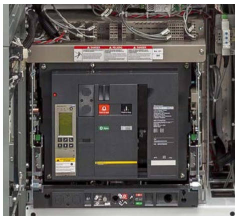
Figure 41 - Breaker Compartment, Door Open
