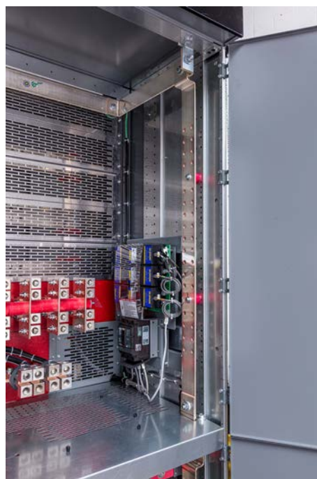
Figure 67 - Surge Protection Device (SPD) in front cable compartment sidewall of Front Accessible PZ-4
