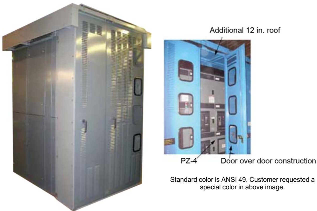
Figure 10 - Indoor Water Resistant Enclosure
