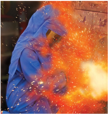
Arc Flash in a Switchboard
