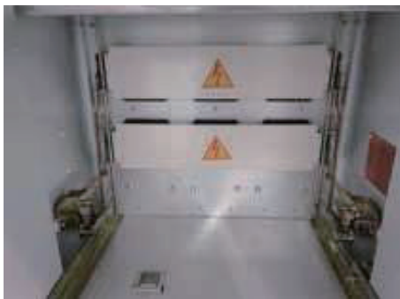
circuit breaker compartment
